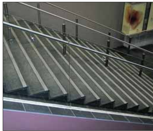
Latham 483 S Asbraloy Mall Bars in stairs at the Conservatorium of Music, Sydney Australia.
