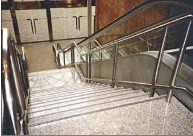
Mall bars inserted in treads.
